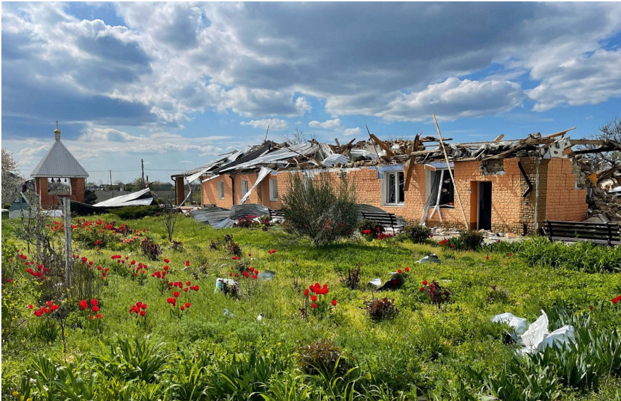
Fig. 1. Ruins of an Orthodox church in the Mykolaiv region (photo: Serhii Belinskyi)
