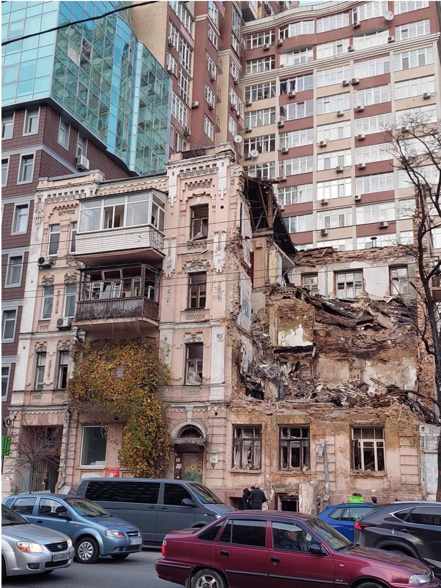
Fig. 8. A house at Kyiv (116a Zhylianska Street) destroyed by a drone hit on October 17, 2022 (photo: Yulia Ivashko)
