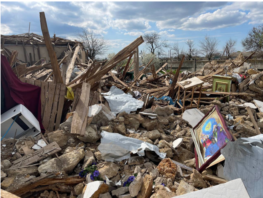
Fig. 2. Ruins of an Orthodox church in the Mykolaiv region (photo: Serhii Belinskyi)
